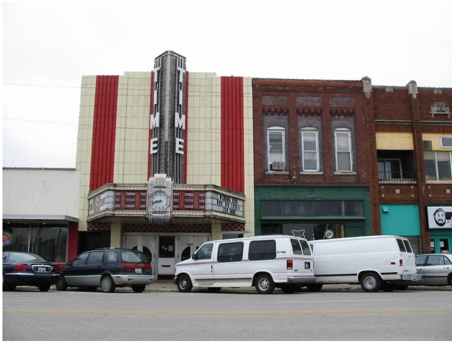
Vacant, Obsolescent, Deteriorated Commercial/Residential
