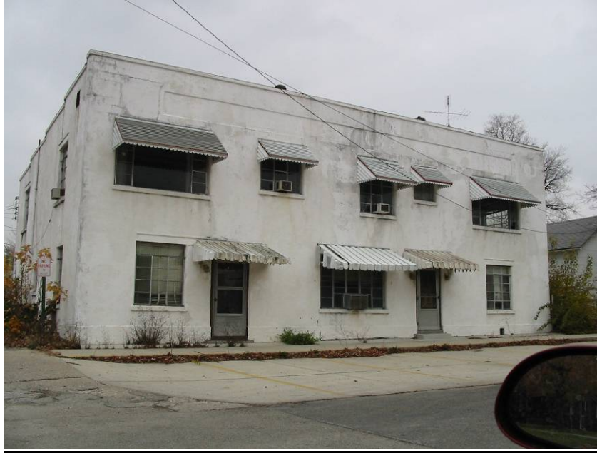
Deteriorated, Dilapidated, Vacant Apartment Building
