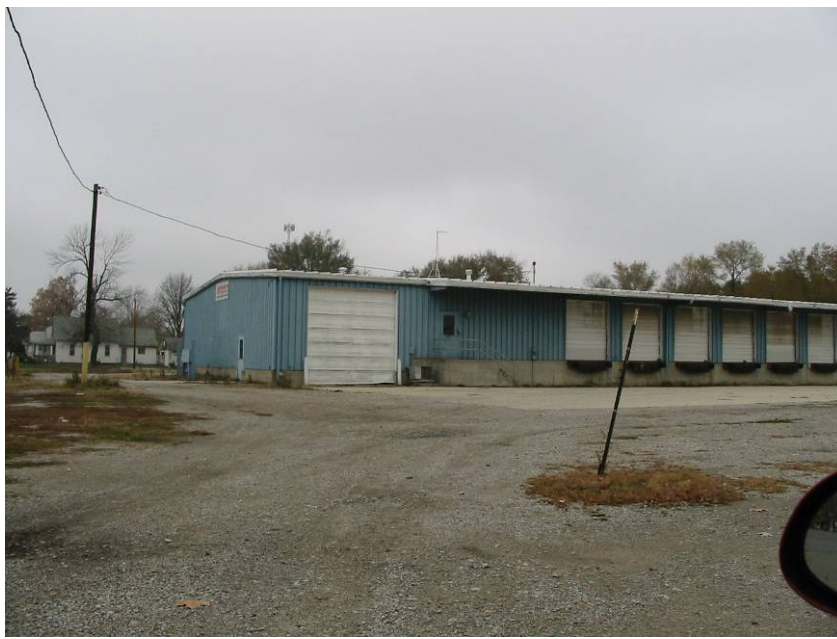
Vacant, Deteriorated Distribution Center
